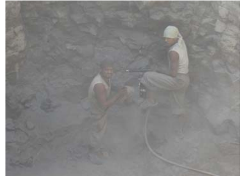
Workers in the new well.
