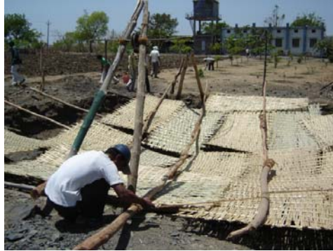
Covering before 2 nd blast
